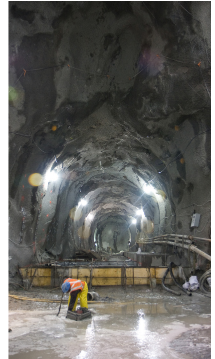
The No. 7 Line Extension Project New York City, New York
